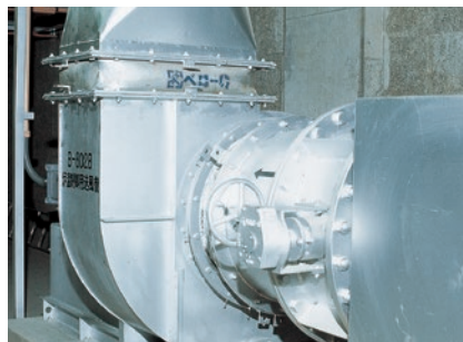
● Bellow-Q™ Non-metallic flexible expansion joint for waste incinerator plants and power plants
